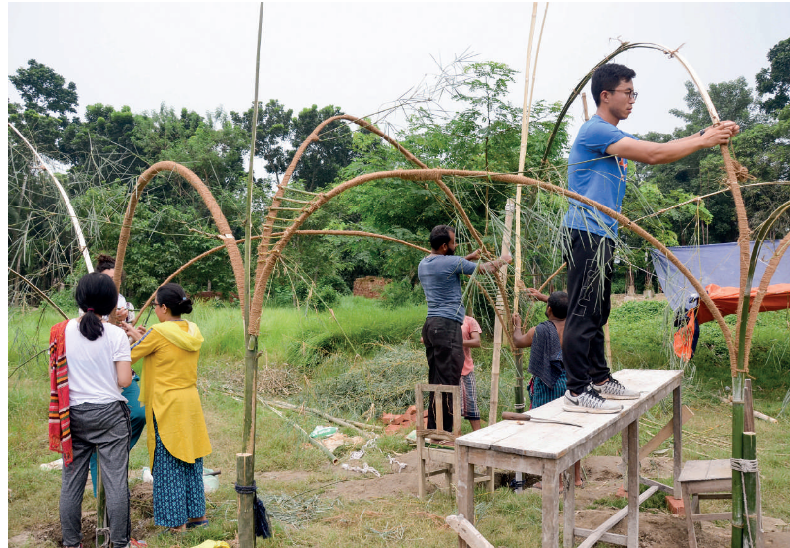
Construction of the Panigram Resort in Jessore, Bangladesh, an eco-resort designed by Tabassum and made from indigenous materials with local labour to promote sustainable tourism. Photo: Marina Tabassum Architects
